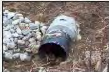
POLYMER LAMINATED CSP RELINE PIPE FULLY BROUGHT
