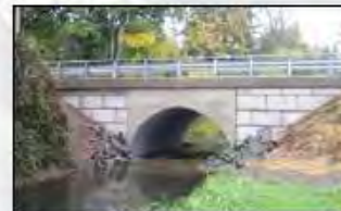
PIPE-ARCH CULVERT WITH BURIED INVERT ON WATERCOURSE
