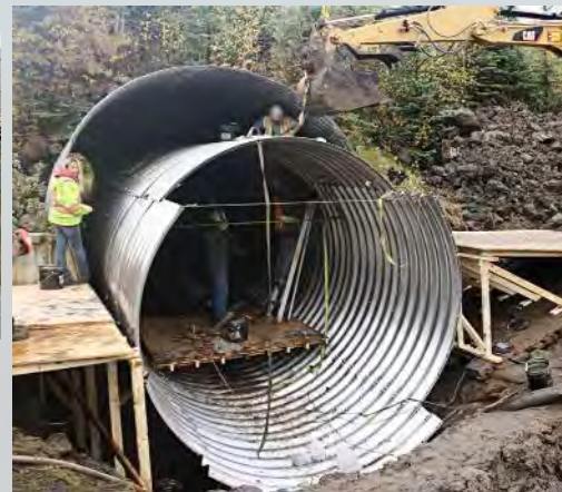
Culvert Rehabilitation
